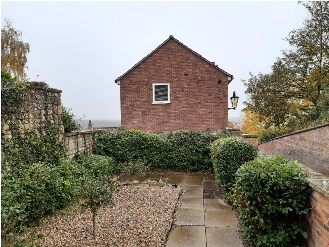
Side elevation of 36 Michaelgate from lower yard, to serve no. 40
